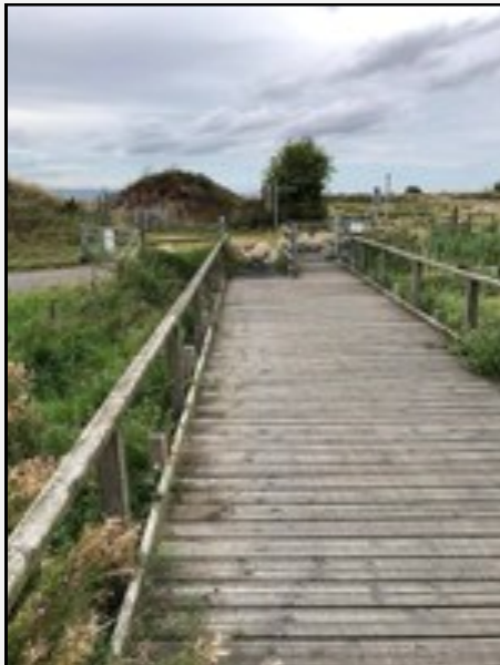
Before (top) and after (below) the repairs
