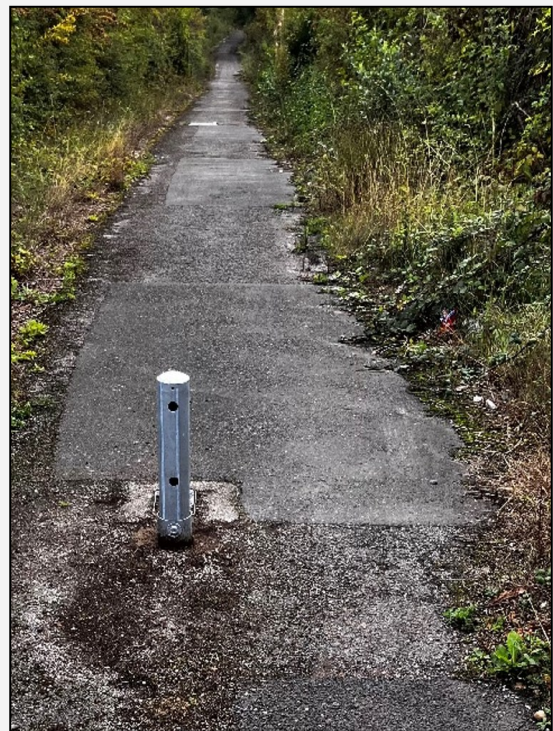
New bollard on Rossmore Road East - looking South but from same point as the previous picture
